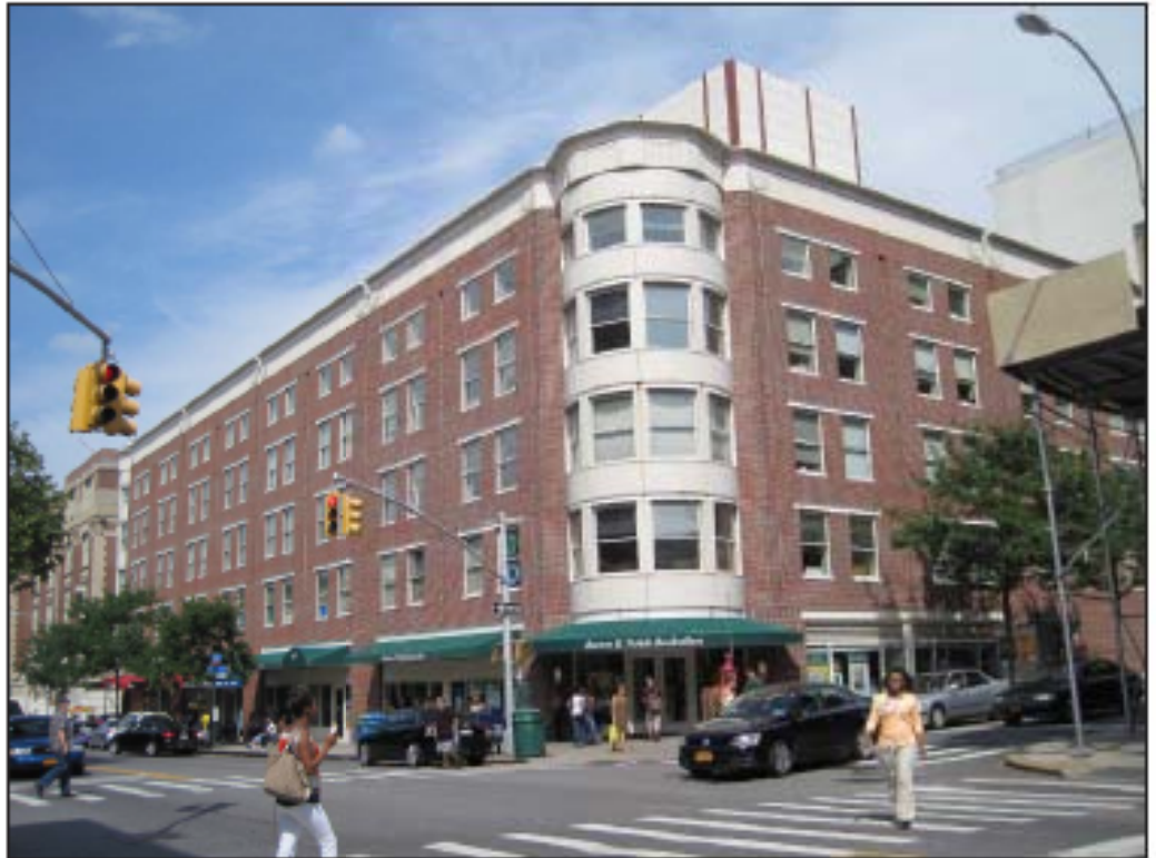
Medical Pavilion. View east on 7th Avenue 7
