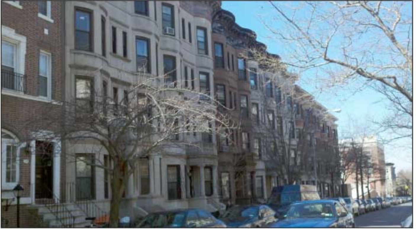
522-532 5th Street, view southwest 17
