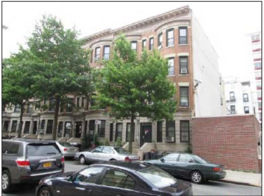
View southeast from 5th Street 6
