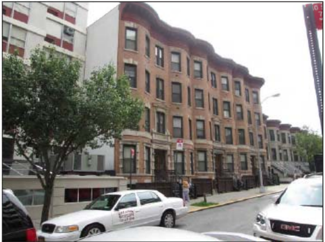
View northeast from 6th Street 8
