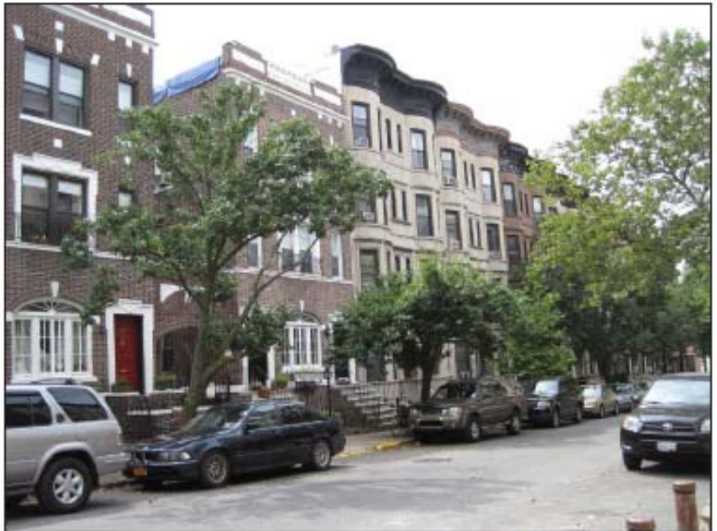
522-540 5th Street. View west 8
