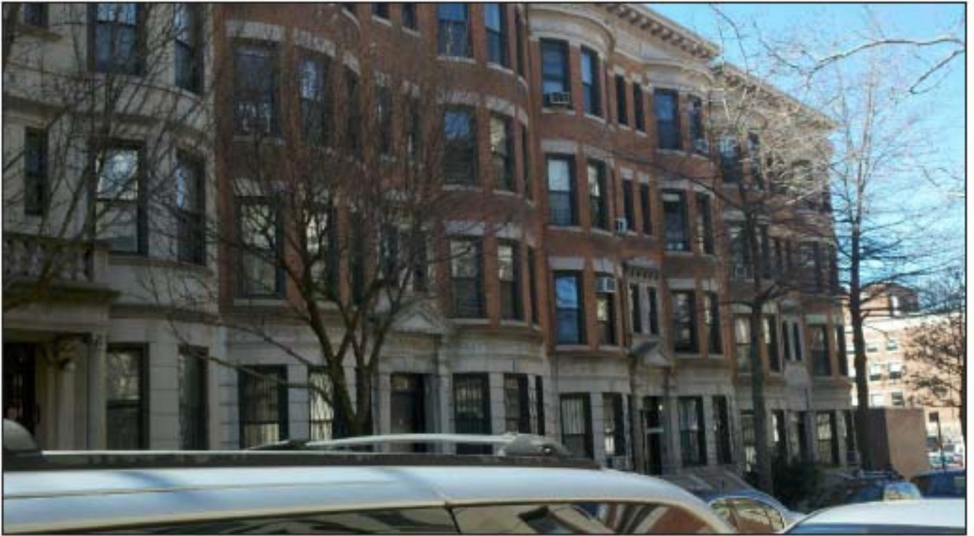
512-520 5th Street, view southwest 3
