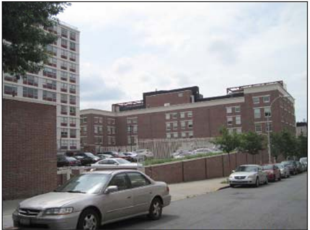
Parking garage. View west on 5th Street 6
