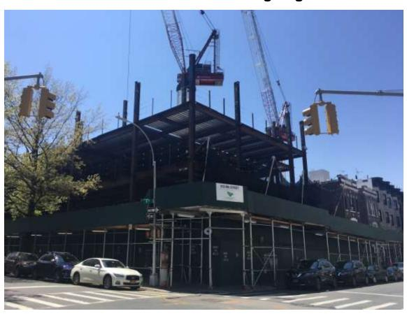
Steel installation is ongoing and both of the tower cranes are operational. As we have shared previously, the arrival of the second crane was delayed due to revisions of the Department of Buildings (DOB) tower crane protocols. The team is working to "close the gap" between the East and the West framing. The logistics on Sixth Street will continue to be implemented and will continue to be extended as needed to accommodate this phase of the project.
