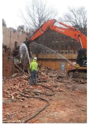
Behind the Fence: A dust control plan is in progress throughout the demolition process. Above: dual hoses are used during the demolition of 510 Eighth Avenue
