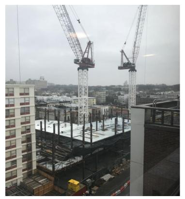
Both of the tower cranes are operational and steel installation is ongoing. As was the case with the first tower crane, the arrival of the second crane was delayed due to revisions of the Department of Buildings (DOB) tower crane protocols. The logistics on Sixth Street will continue to be implemented and will continue to be extended as needed to accommodate this phase of the project.
